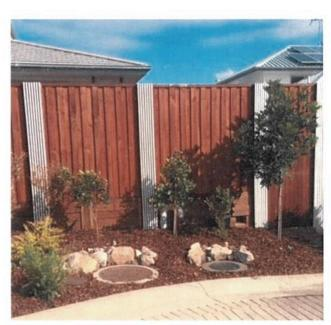
It's important to keep the vacuum pot and valve chamber lids accessible and clear for maintenance.
